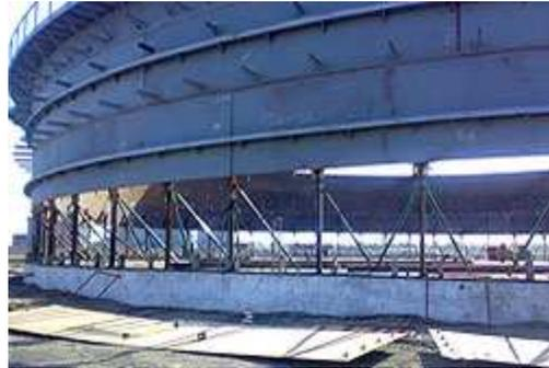
However, with greater emphasis on safety at construction sites, and more stringent quality control, the above method of tank erection did not effectively meet present day requirements. This gave rise to an entirely new concept of erecting the tanks whereby the erection work was restricted close to ground level and the part completed tank was pushed up. The bottom course was erected last.
